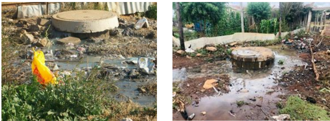
Figure 24: Overflowing bulk sewage points (Photos from Policy Gap 6, 2012)
