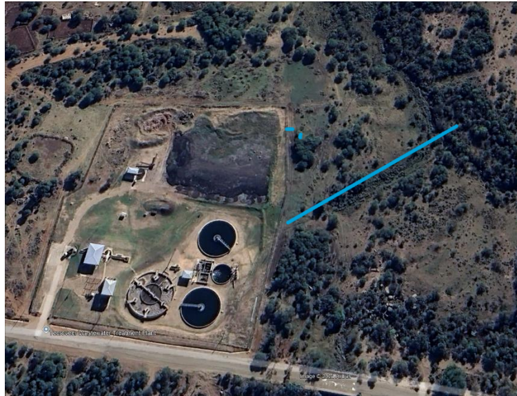
Figure 23: Sewage works from which a canal/stream of condom-laden water flows into the Maretlwane River
